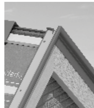
Fig. 27 – Interlock left and right hand trims
