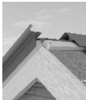
Fig. 26 – Nail left hand trim in place
